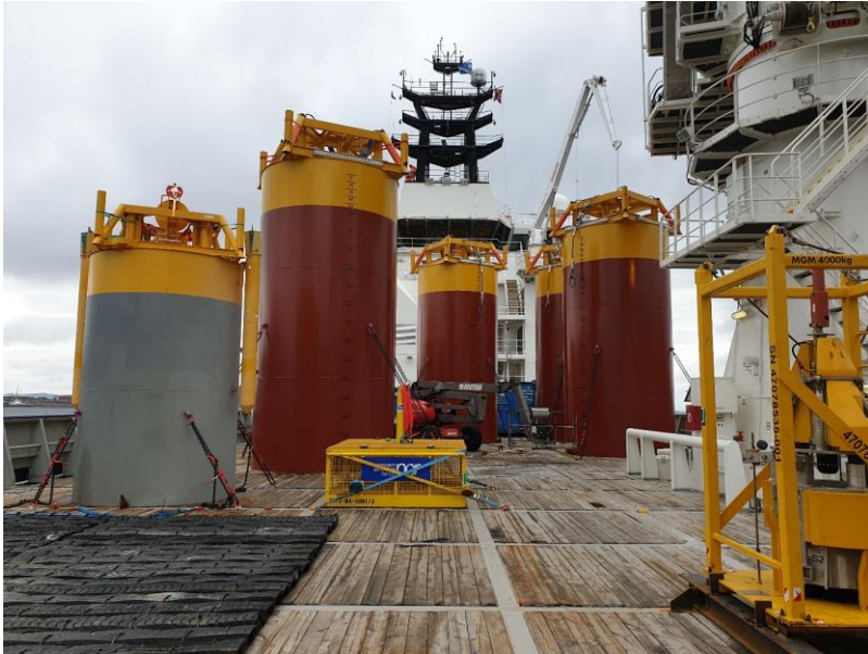
Installation of suction anchors
